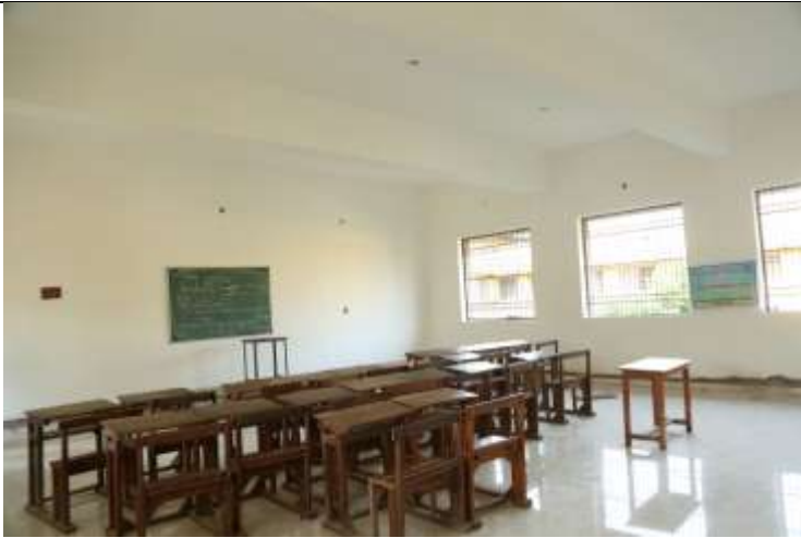
NEW ROOM'S CONSTRUCTED BY RUSA
