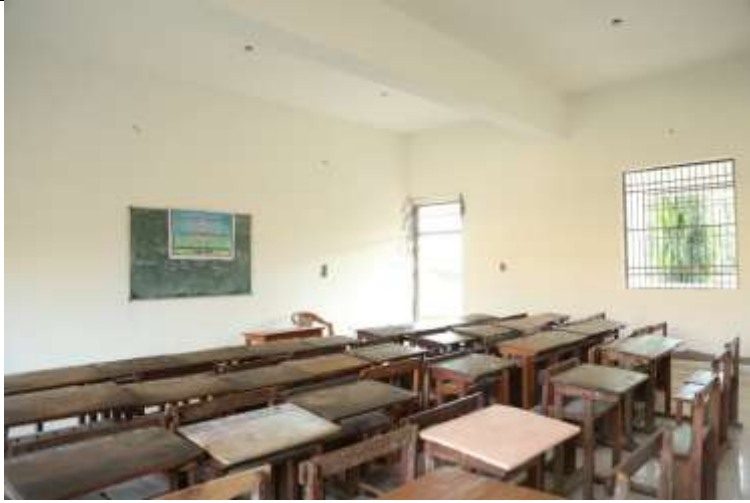
NEW ROOM'S CONSTRUCTED BY RUSA
