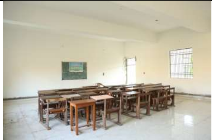
NEW ROOM'S CONSTRUCTED BY RUSA
