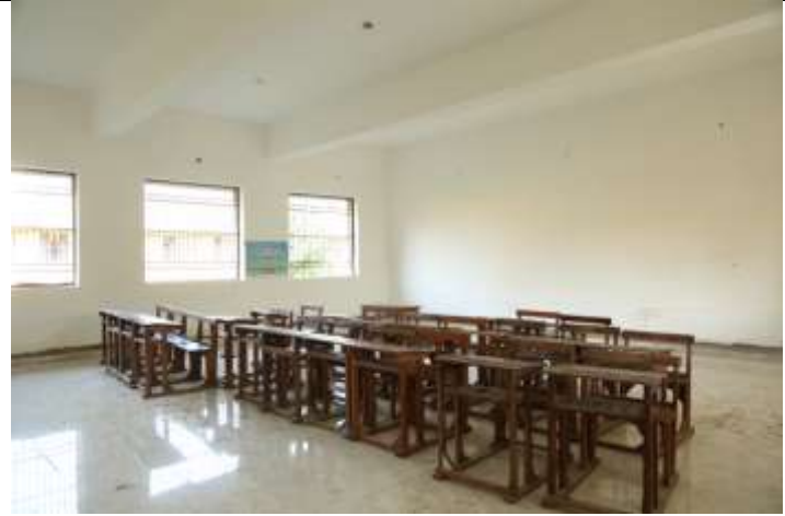
NEW ROOM'S CONSTRUCTED BY RUSA
